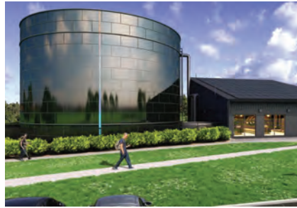
The water battery is helping the university achieve its goal of being carbon-neutral by 2025.
